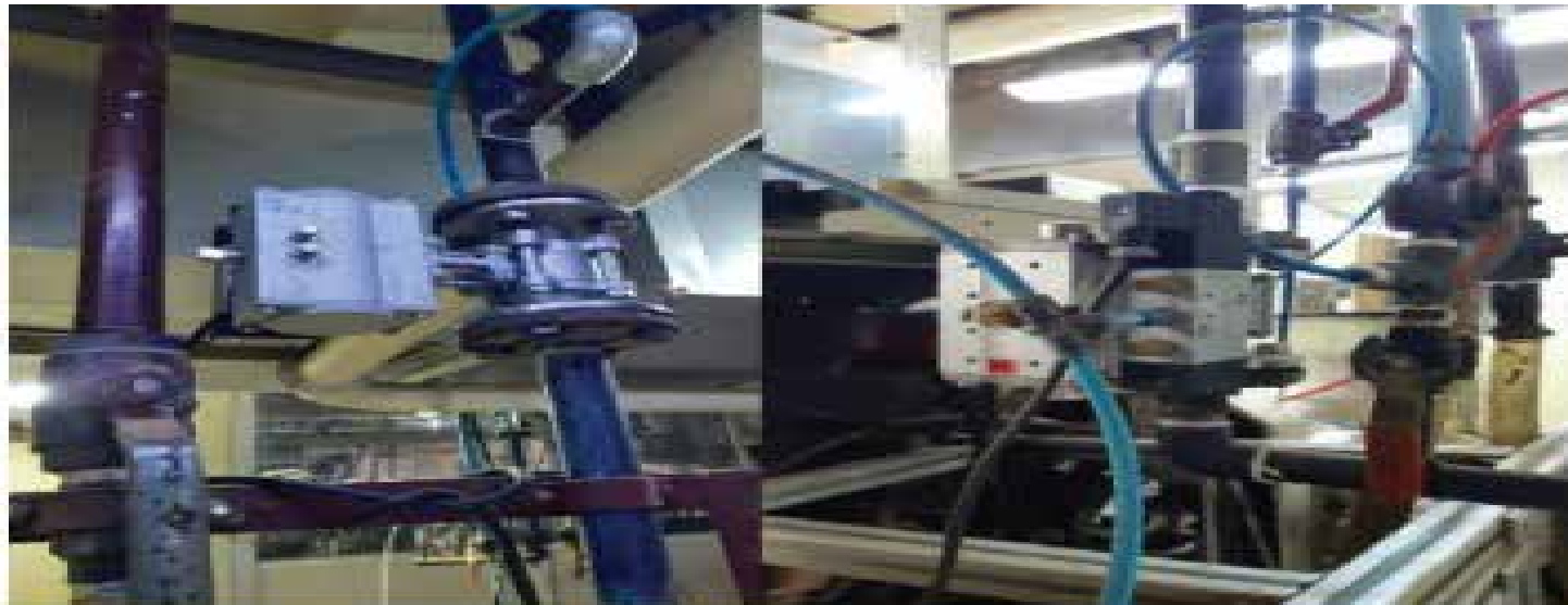
Auto shut off valves on individual machine input of compressed air
